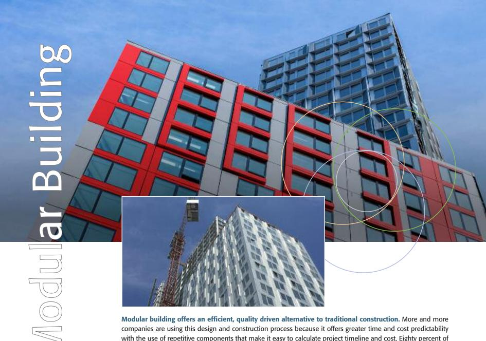
with the use of repetitive components that make it easy to calculate project timeline and cost. Eighty percent of construction occurs off-site resulting in fewer deliveries and reduced neighborhood impact.
